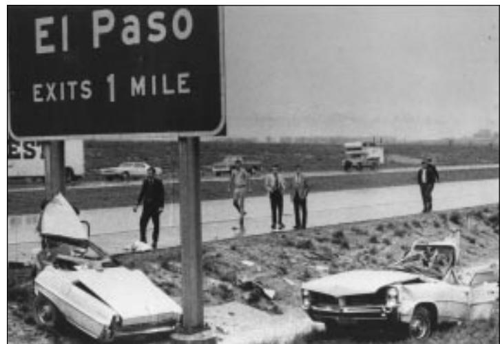
Fig 2 As late as the 1970s newly built highways in the United States had rigid signposts and other roadside hazards, which meant that the consequences of a vehicle hitting one would be severe
